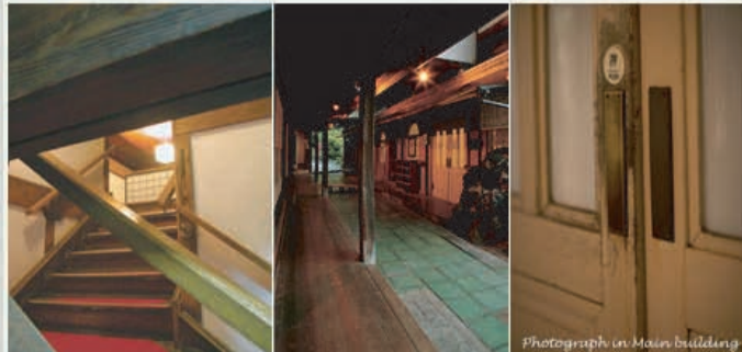
Photograph in Main building
